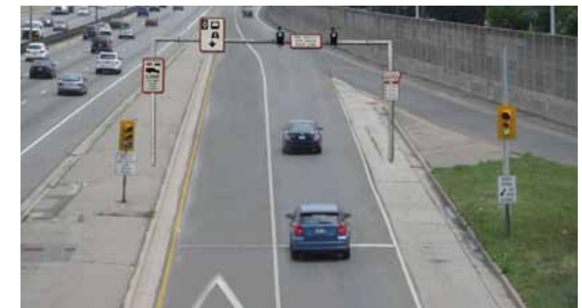
Exhibit 6-2: Examples of Ramp Metering
