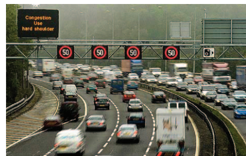
Exhibit 6-6: Examples of Application of Speed Harmonization
