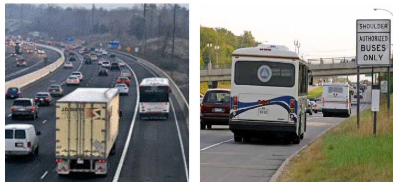
Exhibit 6-3: Examples of Highway Entrance Ramp and Bus Bypass Shoulders
